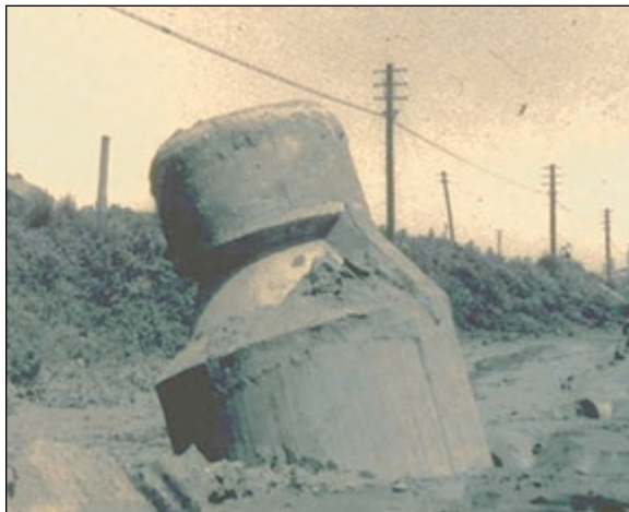
Figure 3-3: Floating manhole, from 1964 earthquake in Niigata, Japan. Damage such as this will be seen following the Seattle Fault scenario earthquake. Photo / NOAA, National Geophysical Data Center
