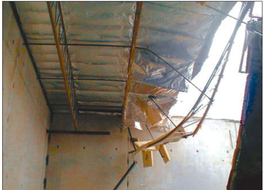
Figure 5-5: Tilt-up building damage, 2001 Nisqually earthquake.
