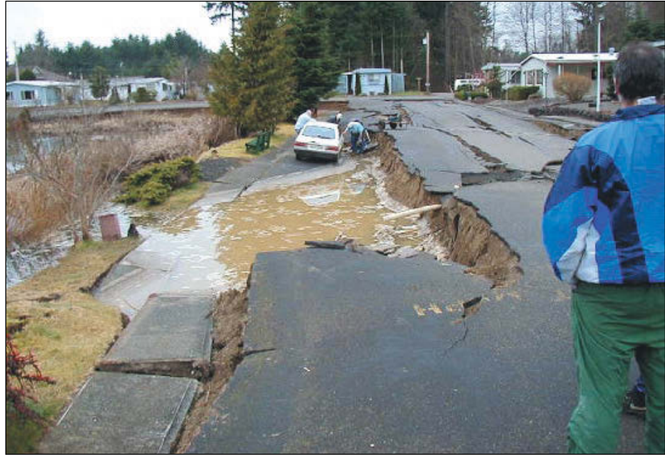
Figure 8-1. A M6.7 earthquake on the Seattle Fault will have impacts region-wide, from business centers to neighborhoods such as this one, whose roads and utilities were extensively damaged by the 2001 Nisqually earthquake.
