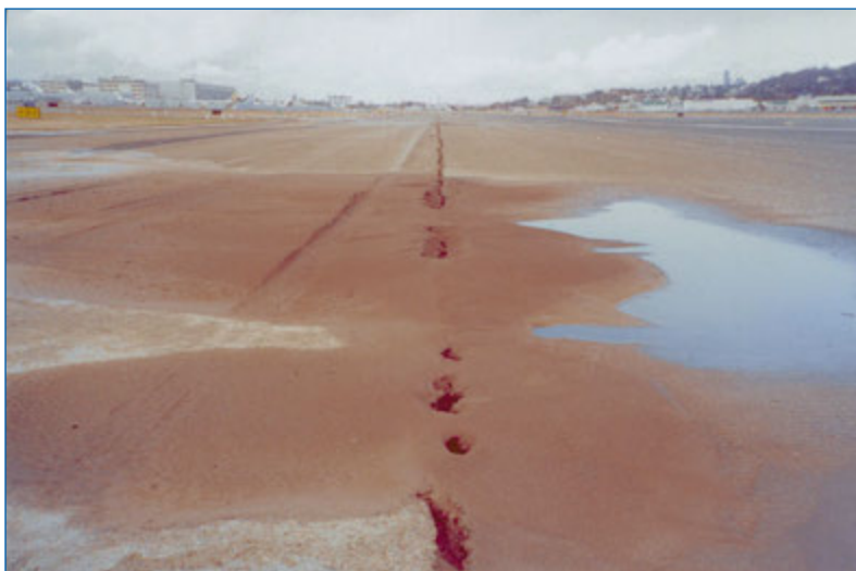
Figure 2-3: Sand boils on the main runway of Boeing Field caused by liquefaction during the 2001 M6.8 Nisqually earthquake.
