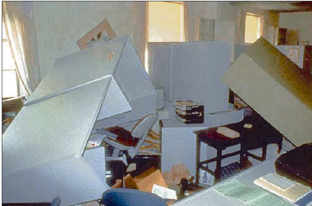
Figure 6-3: Typical nonstructural damage.
