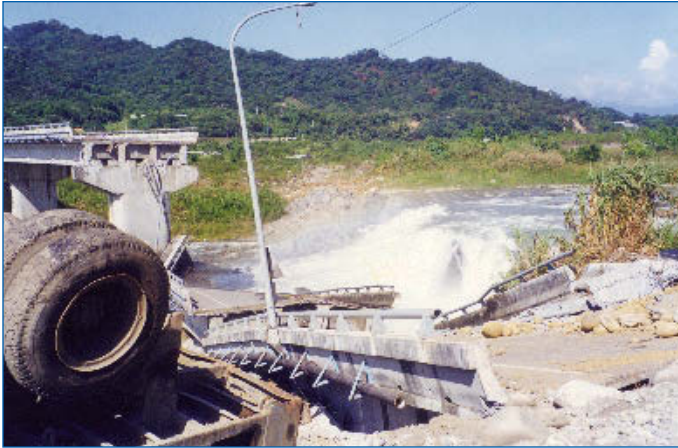
Figure 2-1: In the left photo, surface fault rupture during the Chi-Chi earthquake created a 10 foot waterfall and caused a bridge collapse near Shihkang, Taiwan. In the right photo, we look directly at the fault rupture surface in which the mountains have moved upward approximately 10 feet relative to the coastal plain, lifting and tilting the buildings that straddle the fault.
