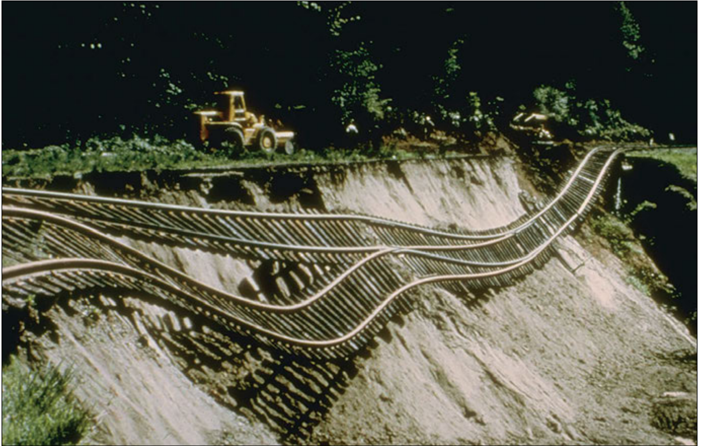
Figure 4-12. Damage to the Union Pacific Railway occurred when hillside fill slid away from beneath a 400-foot section of the branch line just outside Olympia more than 37 miles from the epicenter during the 1965 Puget Sound earthquake.
