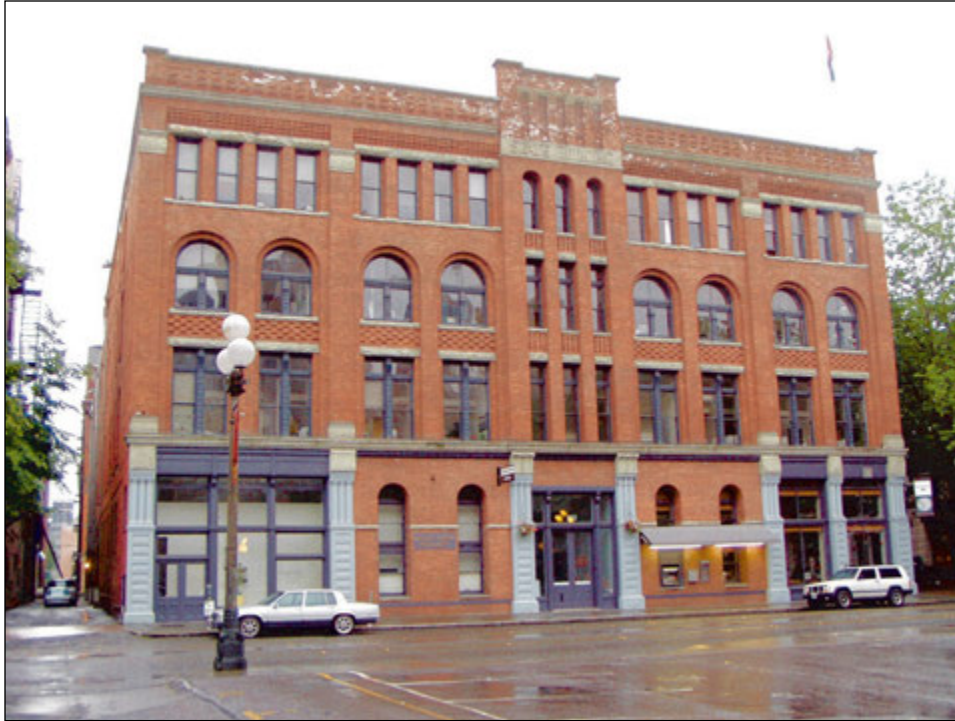
Figure 5-1: A representative unreinforced masonry building in Seattle.
