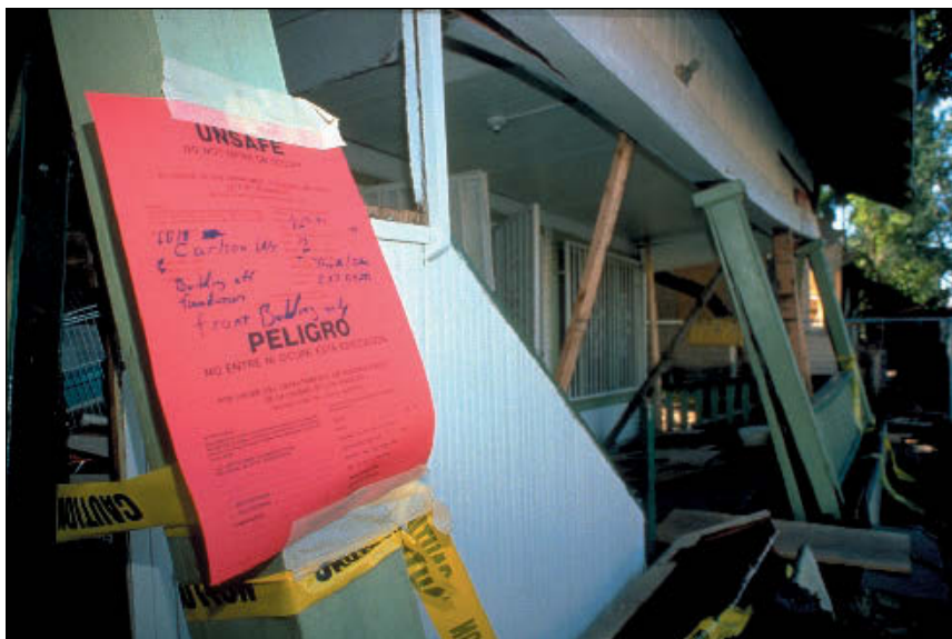
Figure 8-11. Among the activities that will take place immediately after the scenario M6.7 earthquake is inspection of damaged buildings. Those determined to be unsafe will receive a red tag from inspectors.
