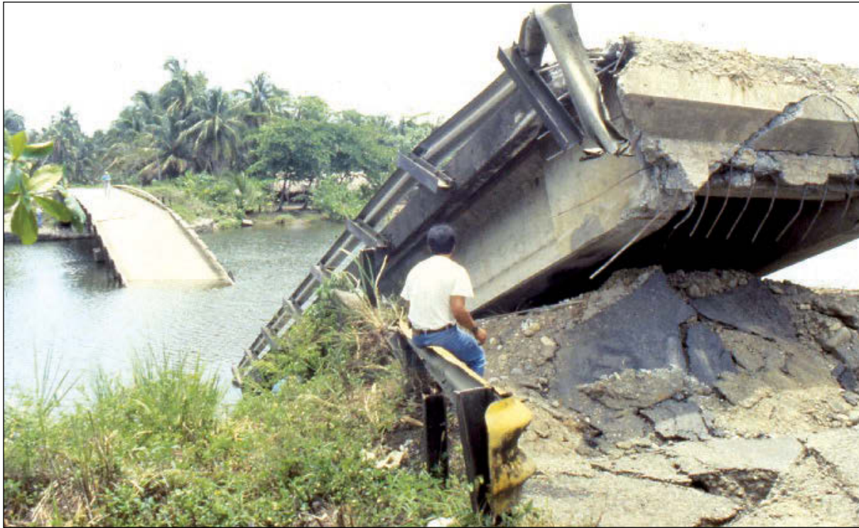
Figure 4-5: Bridge damage from the 1992 Costa Rica earthquake.
