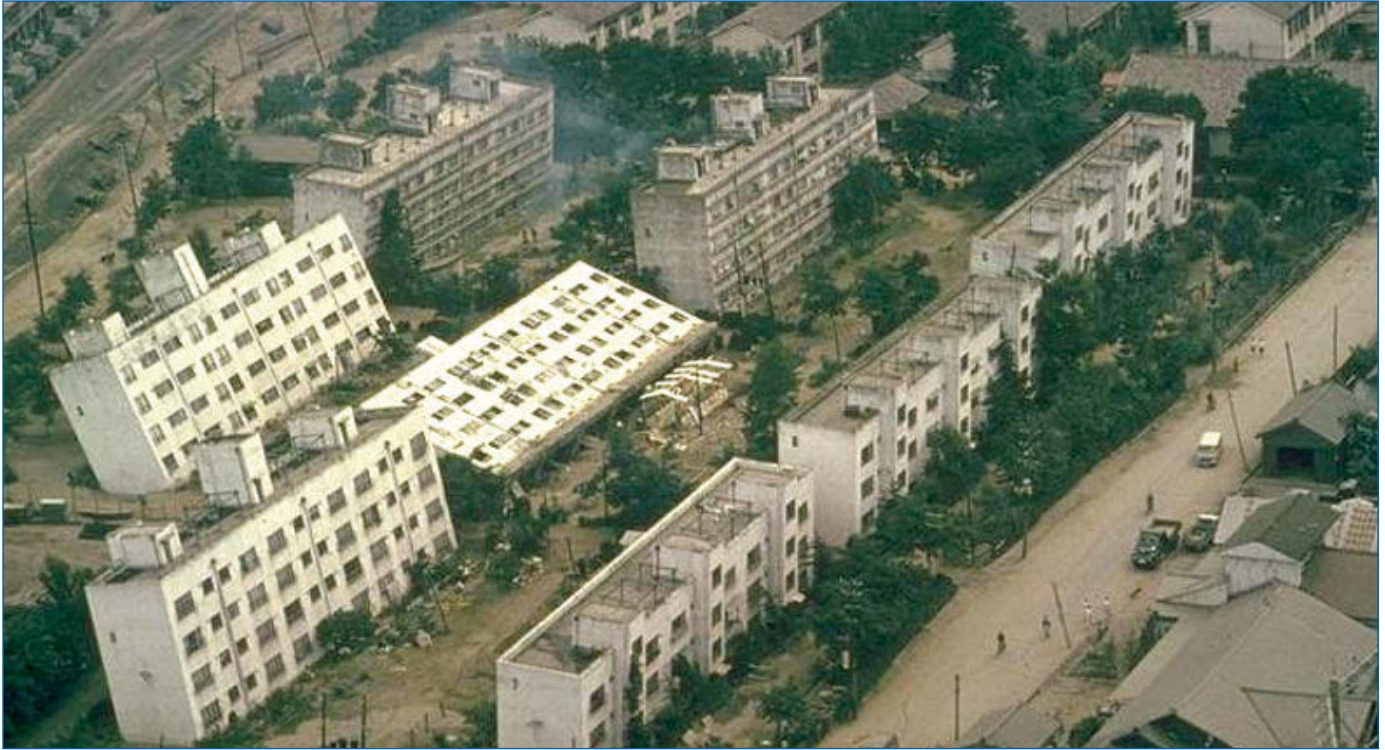
Figure 2-5: Loss of bearing capacity and settlement due to liquefaction during the 1964 Niigata, Japan, earthquake caused these buildings to tip.
