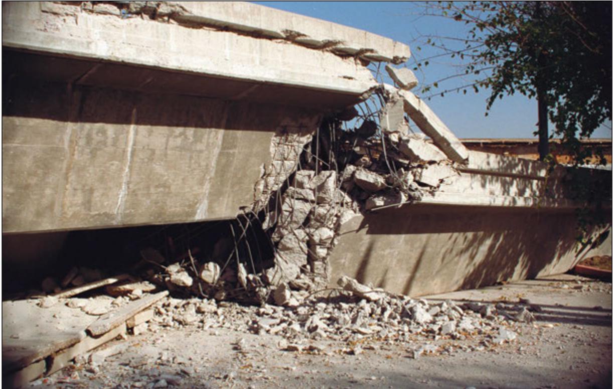
Figure 8-12. The speed with which damage to the transportation infrastructure is repaired will have a direct impact on how quickly the economies of the Central Puget Sound region and the state recover following the scenario earthquake.
