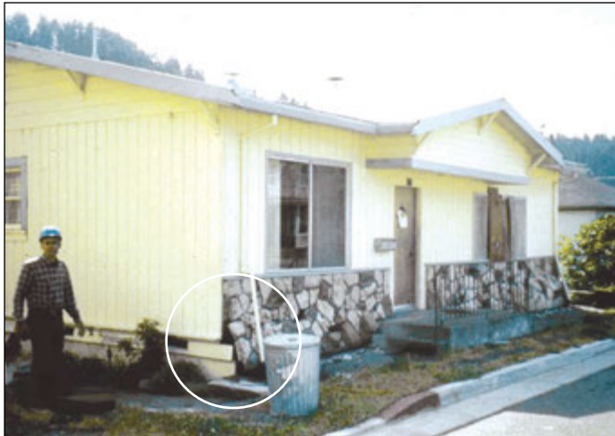
Figure 5-10: Example of residential damage expected in the scenario earthquake. Homes not bolted to their foundations can be shaken off them by strong ground shaking (see damage inside white circle). Photo / Applied Technology Council
