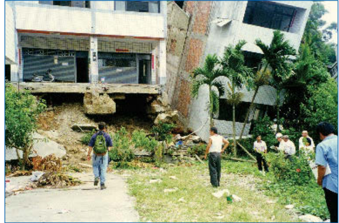
Figure 2-1: In the left photo, surface fault rupture during the Chi-Chi earthquake created a 10 foot waterfall and caused a bridge collapse near Shihkang, Taiwan. In the right photo, we look directly at the fault rupture surface in which the mountains have moved upward approximately 10 feet relative to the coastal plain, lifting and tilting the buildings that straddle the fault.
