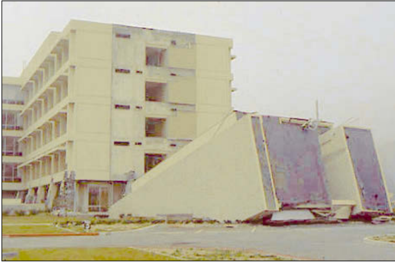
Figure 6-2: Olive View Hospital. Built before the 1971 Sylmar, CA earthquake, it was constructed with non-ductile concrete frames and shear walls vulnerable to ground shaking damage.
