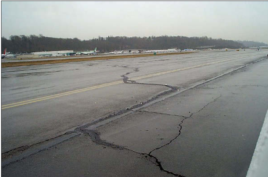
Figure 4-9: Long cracks and liquefaction at King County International Airport runway, commonly known as Boeing Field.
