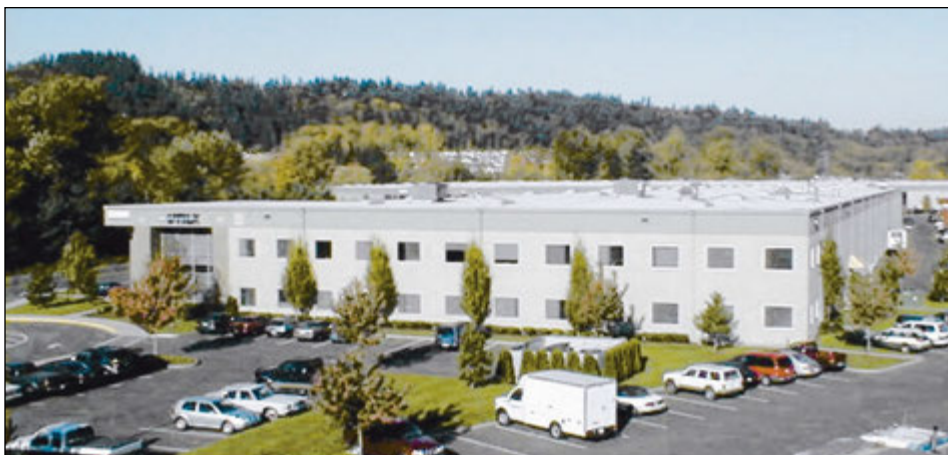
Figure 5-4: Example tilt-up building in Seattle.
