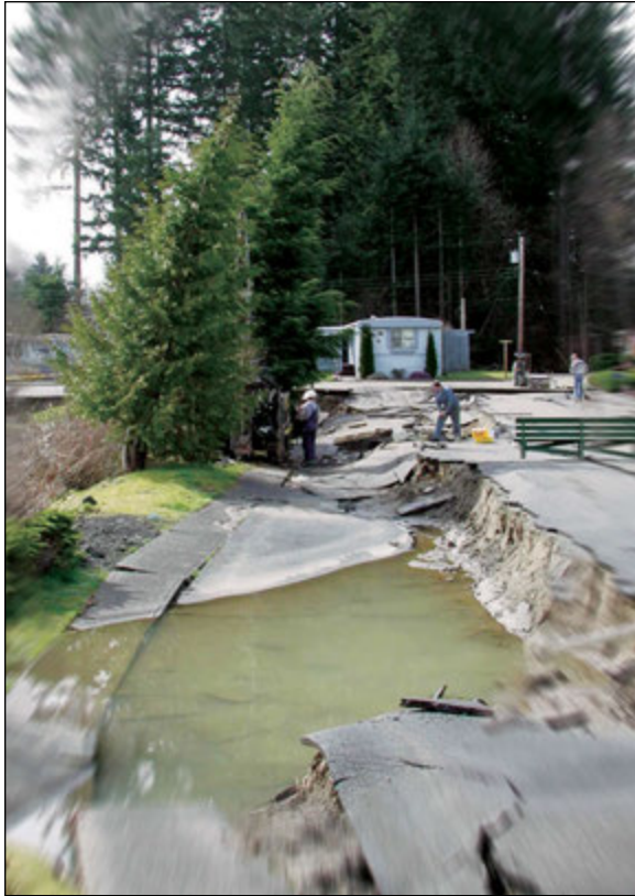
Figure E-1: Damage to roads, similar to what this Tumwater neighborhood experienced in the 2001 Nisqually earthquake, will be widespread throughout the region close to the rupture in the scenario Seattle Fault earthquake.
