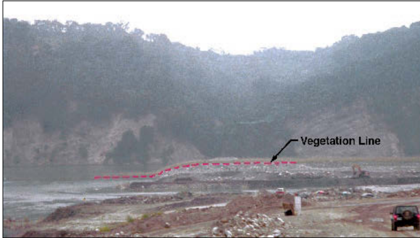
Figure 2-2: The vegetation line across the middle of the photo shows the original ground surface. Fault rupture during the Chi-Chi earthquake raised the ground and river channel on the right hand side of the photo, causing flooding upstream.
