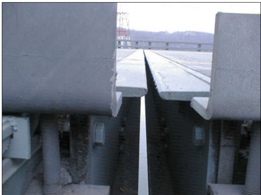
Figure 4-6: Moveable bridge alignment problems after Nisqually earthquake.
