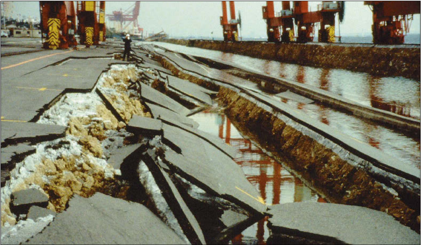
Figure 4-11: Damaged quay walls and port facilities on Rokko Island from the 1995 Kobe earthquake. Quay walls were pushed outward by 6.5 to 10 feet, with 10- to 13-foot-deep depressed areas called grabens forming behind the walls.
