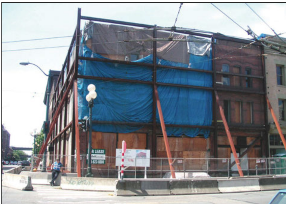
Figure 5-2: Unreinforced masonry building damage, 2001 Nisqually earthquake.
