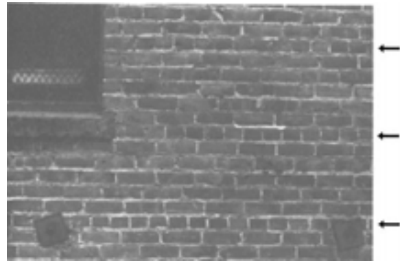
Figure D-10 URM wall showing header courses (identified by arrows) and two washer plates indicating wall anchors.
