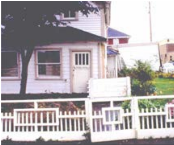
Figure F-10 This house has settled to the ground due to collapse of its post and pier foundation.
