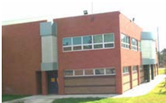
Figure E-46 Modern reinforced brick masonry.
