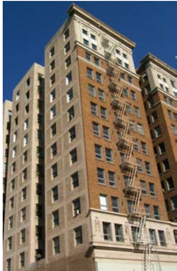
Figure 5-9 Exterior view of 3711 Roxbury.
