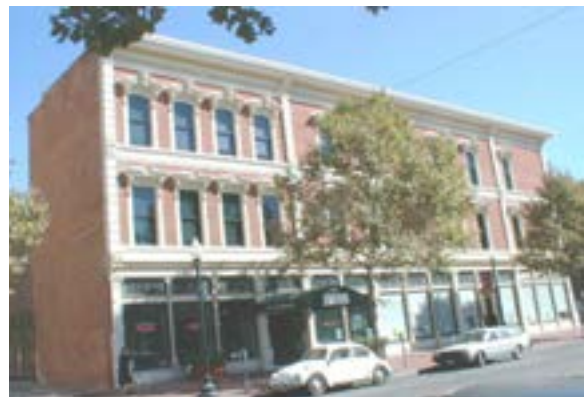
Figure E-51 West coast URM bearing-wall building.
