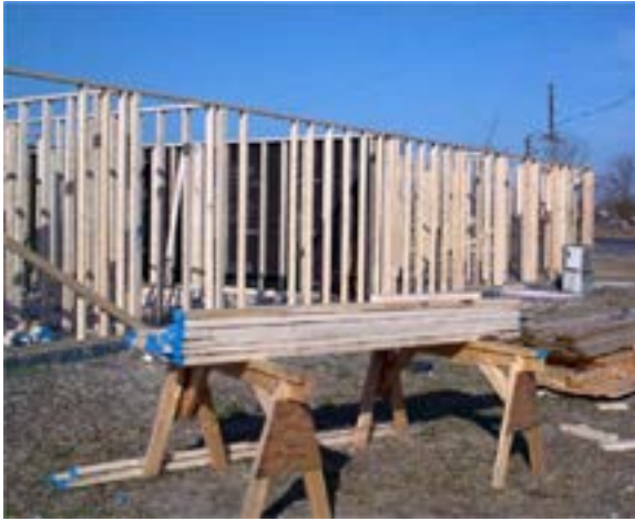
Figure E-4 Stud wall, wood-framed house.
