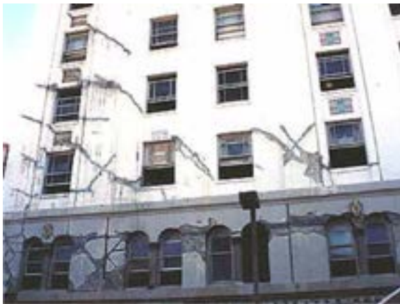
Figure E-32 Shear-wall damage, 1989 Loma Prieta earthquake.
