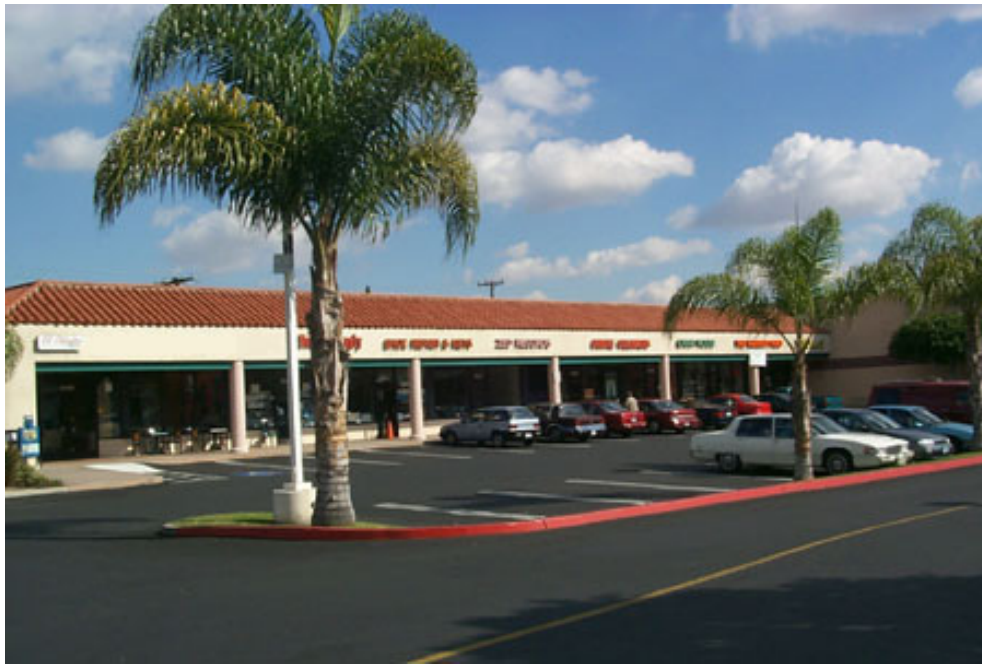
Figure 5-14 Exterior view of 1450 Addison Avenue.
