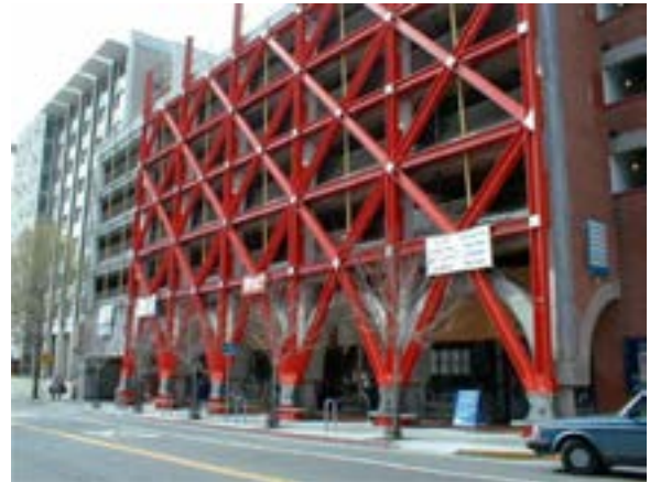
Figure E-15 Rehabilitation of a concrete parking structure using exterior X-braced steel frames.
