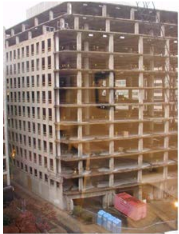
b. Reinforced concrete frame under renovation – demolition of older facade units.
