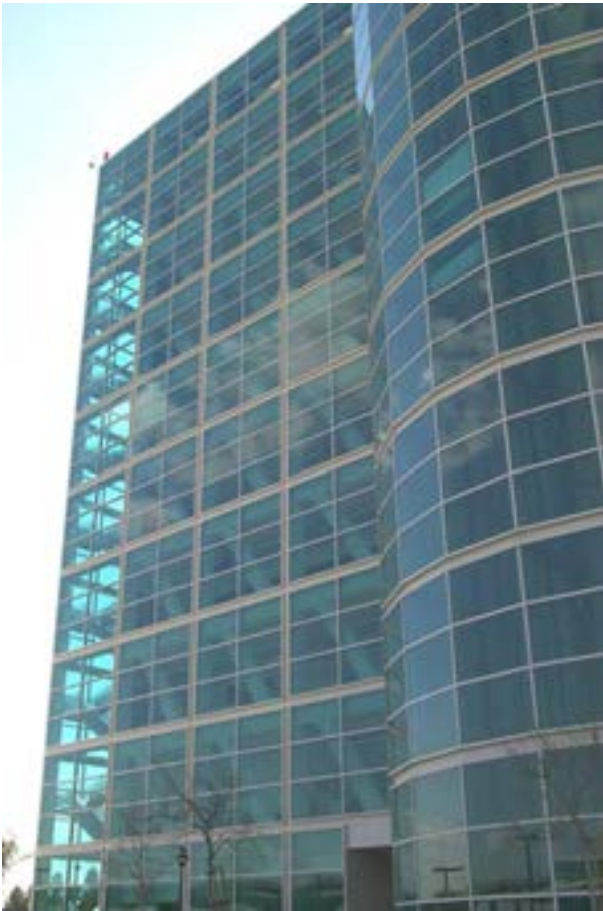
Figure 5-5 Exterior view of 3703 Roxbury Street.
