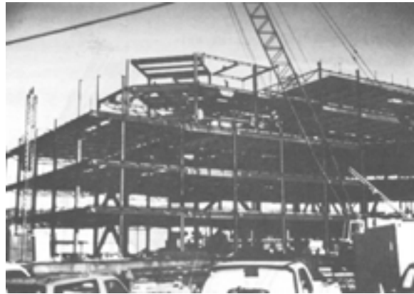
Figure E-13 Braced steel frame, with chevron and diagonal braces. The braces and steel frames are usually covered by finish material after the steel is erected.
