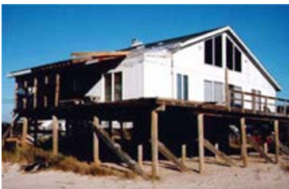
Figure E-6 Timber pole framed house.
