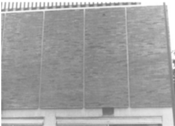
Figure D-13 Brick veneer panels.
