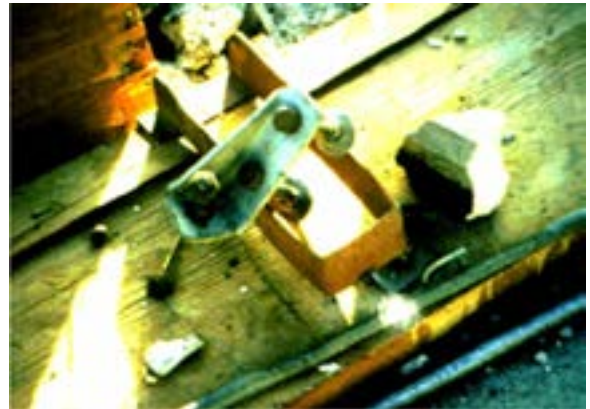
Figure E-38 Tilt-up construction anchorage failure.
