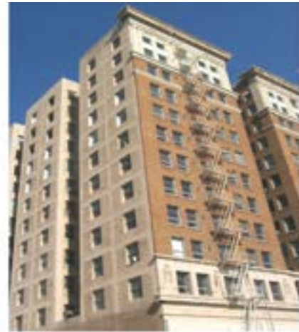
Figure E-33 Concrete frame with URM infill.
