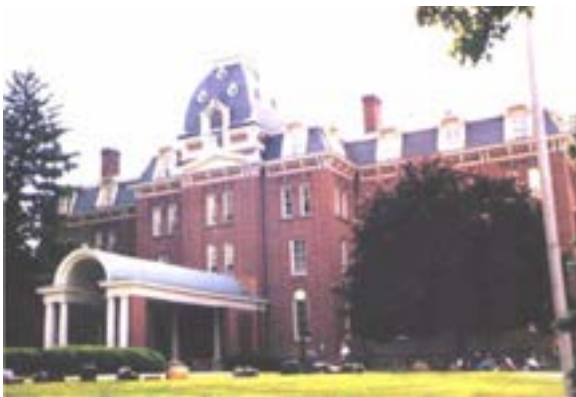
Figure E-50 East coast URM bearing-wall building.
