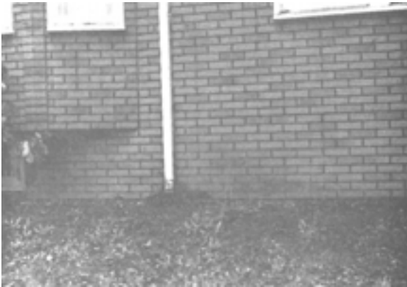
Figure D-16 Asphalt siding with brick pattern.
