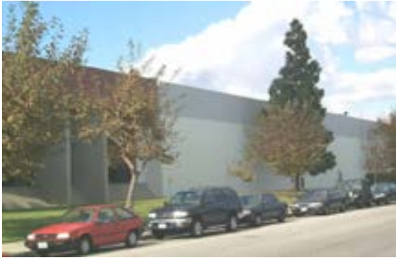
Figure E-36 Tilt-up industrial building, 1970s.
